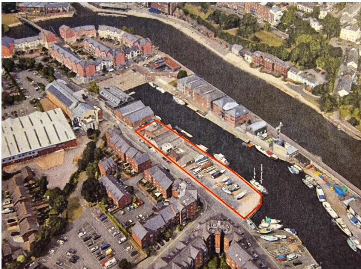
Aerial view of Exeter Canalside (site boundary shown in red)
